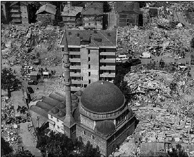
Figure 2: An image from Enric Marti of the Associated Press that was taken for the New York Times on August. "A mosque stood with a few other structures amid the rubble of collapsed buildings in the town of Golcuk 60 miles east of Istanbul". [ http://arrowsmith510.asu.edu/Ex-ercises/Exercise3/ ]
