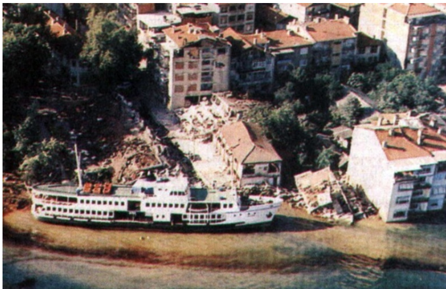
Figure 5. Damage from the earthquake 1999, tectonic subsidence, ground liquification and the tsunami. The ship in the foreground thrown onshore by tsunami wave action. [Kandilli Observatory and Research Institute, [www.drgeorgepc.com/ Tsunami1999Turkey.html, accessed on 14.04.08]
