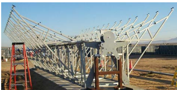
Figure 3: Space frame of a EuroTrough module with measurement targets on the mirror support points
