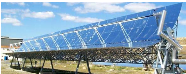
Figure 2: EuroTrough line focussing collector module
