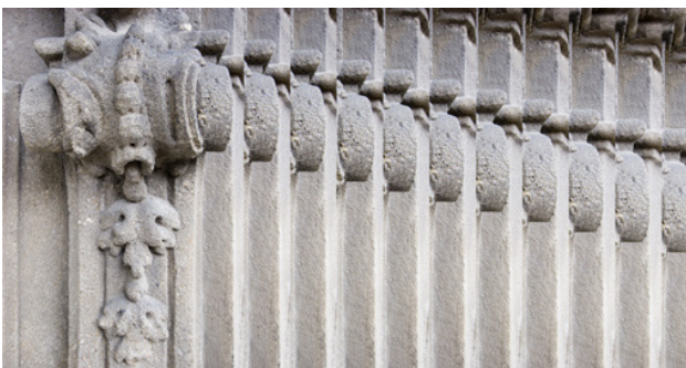
Figure 2. Images taken by moving camera
