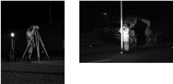
Figure 4. Precise levelling of reference points on the viaduct.
