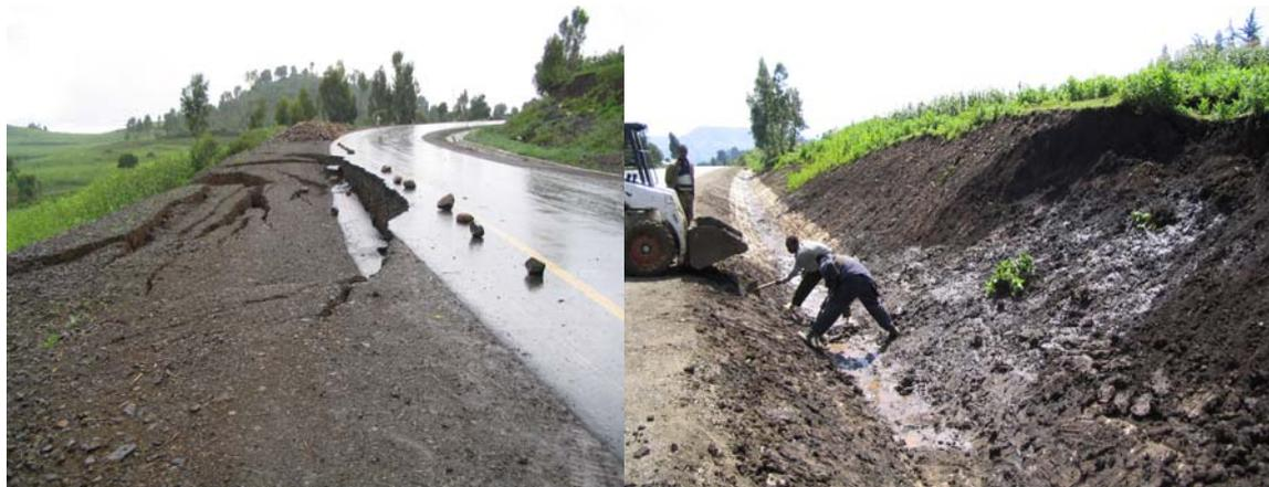
Figure 1. Failure of road pavement due to presence of exposed expansive soils beneath the side slope of road embankment (left), road side drain or ditch clogging due to slumping of expansive soil from bare back slope (right).
