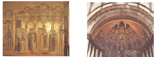
Figure 1. The San Marco Basilica’s domes before (left) and after (right) building of superstructures in wood and lead
