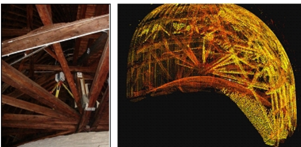
Figure 2. On the left, a picture taken during scanning at the second level of the “Pentecoste” dome; on the right, the point-cloud made up of the 18 scans captured at 3 different levels.
