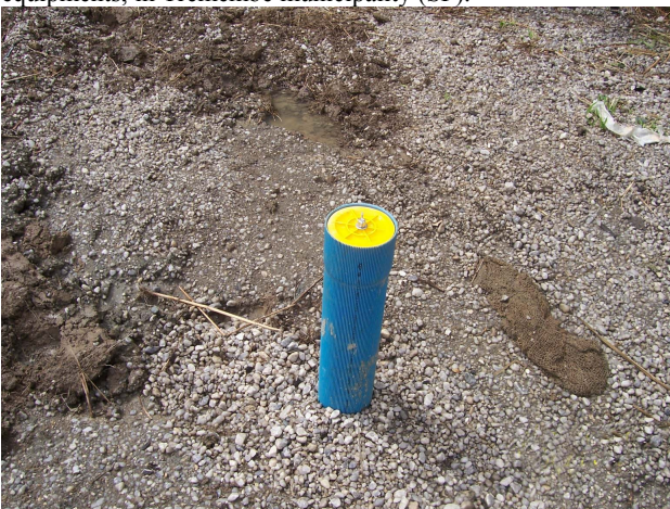
Fig. 11- A piezometer installed in Tremembé municipality (SP)
