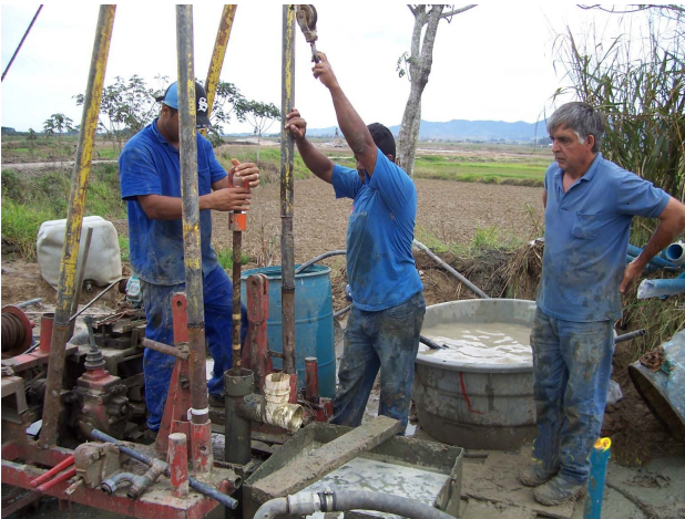
Fig. 10- Activities in the installation of data collection equipments, in Tremembé municipality (SP).
