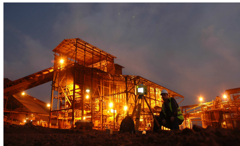
Fig 2 - View of a part of the refinery during the survey
