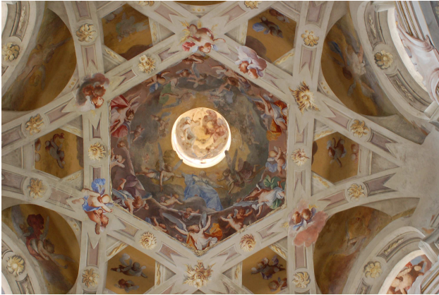
Fig 3 - The spectacular dome from the inside
