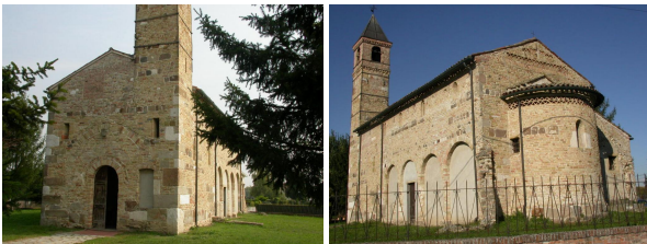
Figure 7: Two views of the Pozzoveggiani church.
