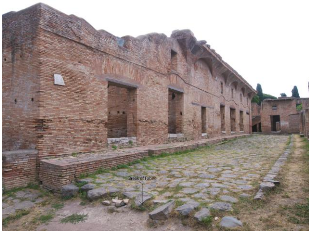
Fig. 16 Break on the surface of the Via di Balconi
