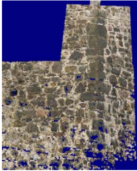
Figure 7. Close-up of a wall corner part
