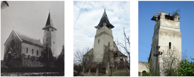
Figure 10. Banostor church – Old photo, 4 years ago and today
