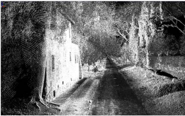
Figure 15: Appian Way Historical Building
