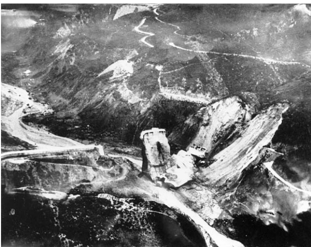
Figure 2: The St Francis Dam after failure, looking east. Note the central "Tombstone" remnant of the dam wall and the landslide scarp on the right-hand side of the image (Courtesy of Santa Clarita Valley Historical Society/SVCHISTORY.com).
