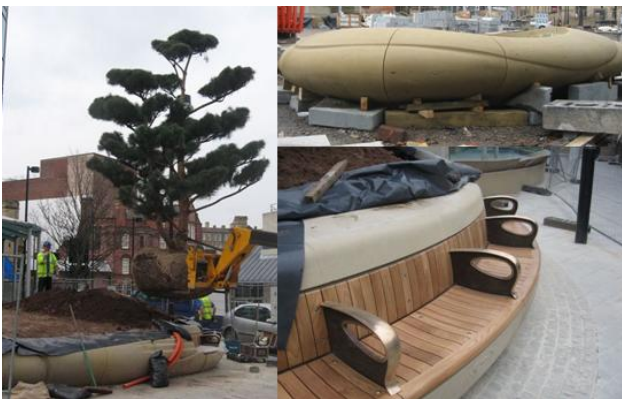
Figure 11. On-site installation of the planters in Tudor Square.
