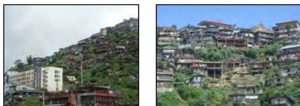
Figure 2. Urban Sprawl along the Slopes of Baguio City (LCVerzosa, 2009)
