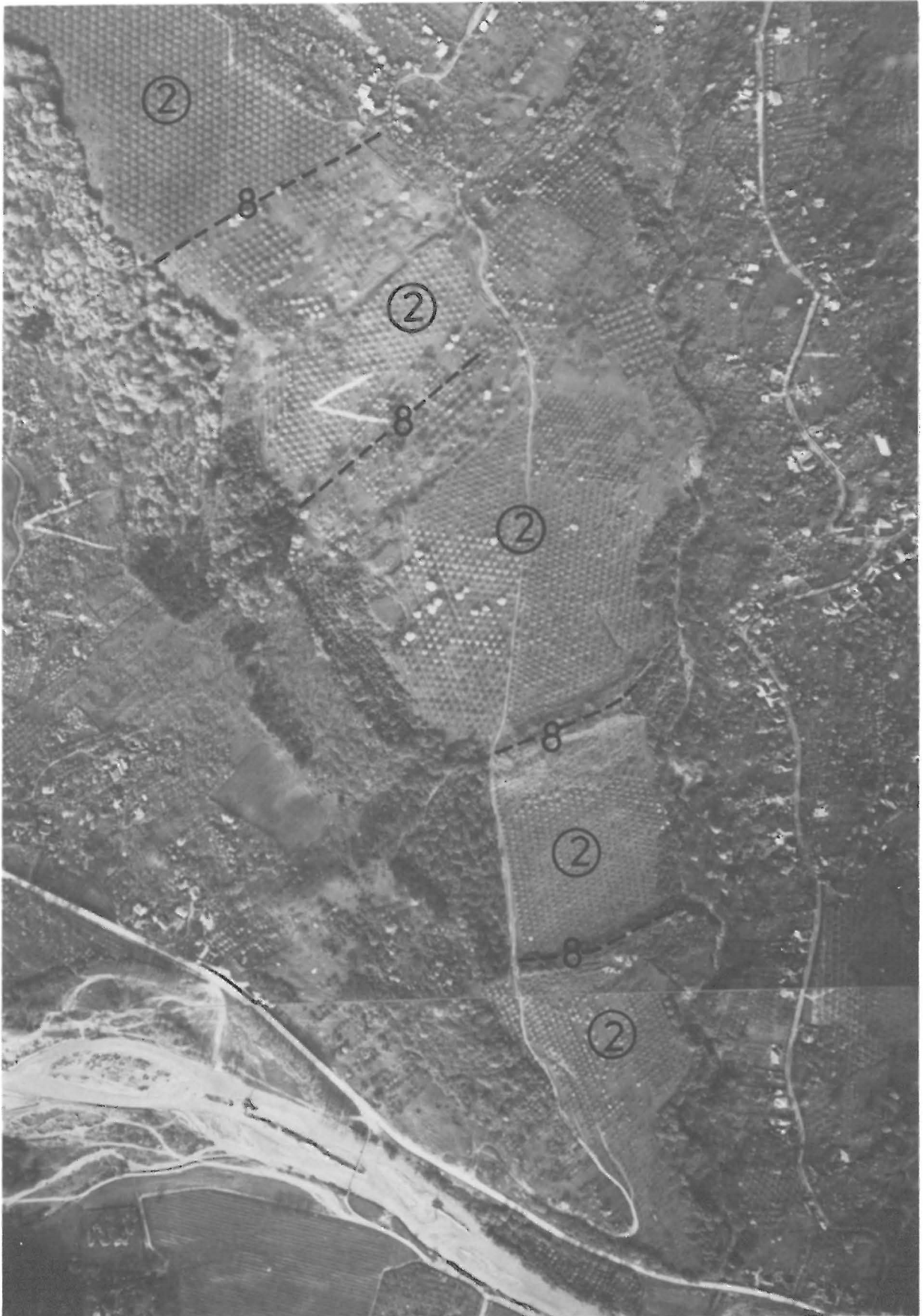
Fig.2 Aerial photograph showing the situation of the area in 1978 (before the sliding)
