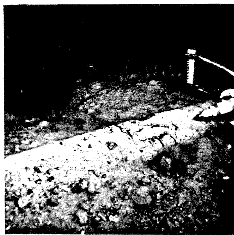
FIG 4. Underwater photograph of damaged pipe
