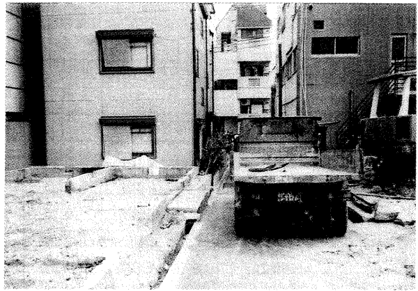
Photograph 3. Fireproof Building (Nada District)
