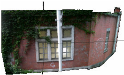
(b) Left side of a building
