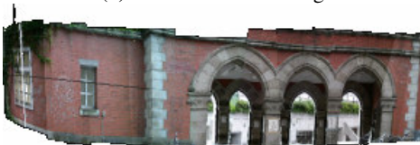
(c) Front side of a building
