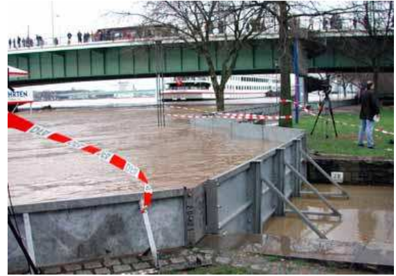
Figure 7: Mobile wall in the city of Cologne †
