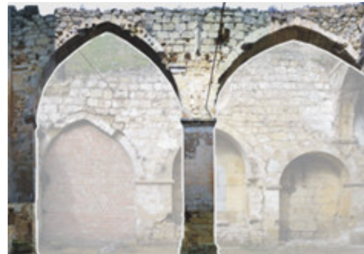
Figure 12. Images rectified mosaic of rear arches in the nave
