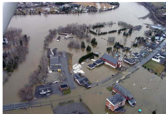
Figure 2. Flooding of St. John River in 2008
