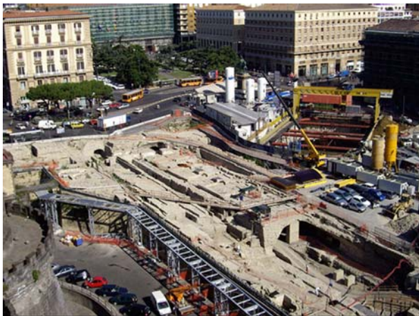
Figure 1. Overview of the site, july 2006
