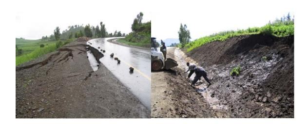
Figure 1. Failure of road pavement due to presence of exposed expansive soils beneath the side slope of road embankment (left), road side drain or ditch clogging due to slumping of expansive soil from bare back slope (right).
