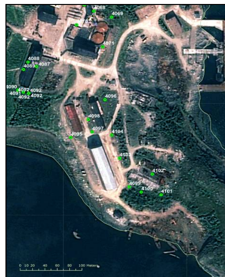
Figure 12. Location of boreholes drilled as part of the survey of the contaminated site area around Building 5, the DSU and the SRW storage facility
