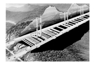
Figure 2. Ventilation System of Hsueh-Shan Tunnel
