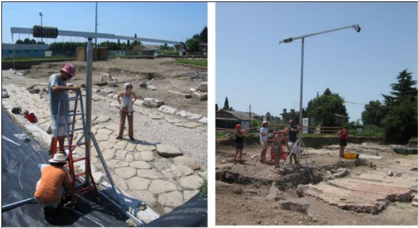
Figure 2 . Assembly and raising pole on site.
