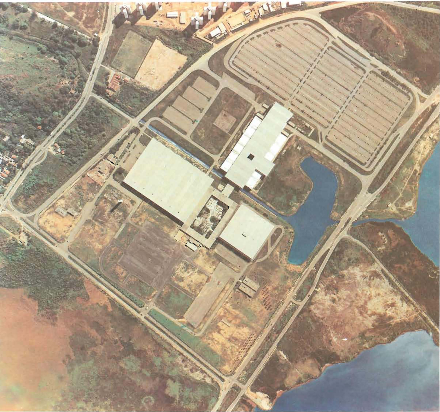
The Rio Center, site of the 1984 ISPRS Congress (made available by Aerofoto Cruzeiro)
