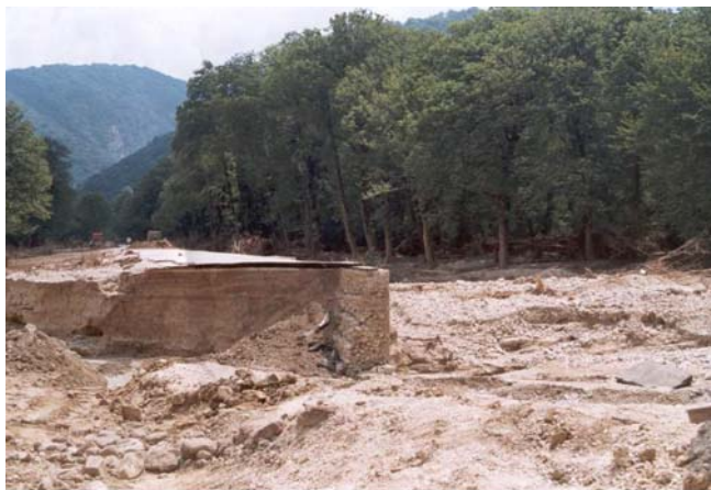
Figure 4: to surge flood in GOLESTAN province
