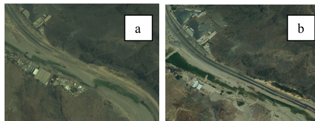
Figure 8. Main road connecting Muscat and Qurayat (a) after Gonu and (b) after Phet
