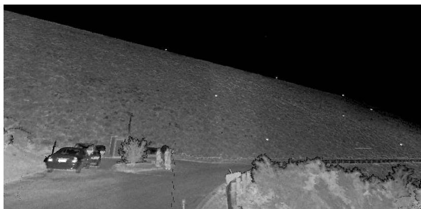
Figure 3. North Dandalup Dam Scanner Image
