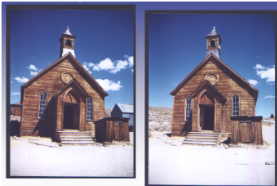
Figure 3. Photographs of Bodie's Methodist Church.
