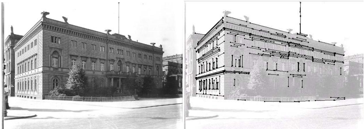
Figure 2. The Meydenbauer image (left) and the automatically extracted image lines (right).
