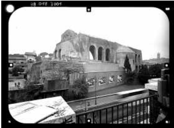
Fig. 3: Metric image of the north-east side of the basilica
