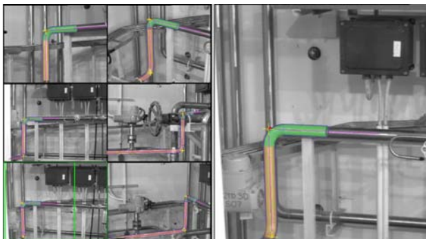
Figure 8. Construction of a piping component
