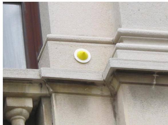
Figure 6. A target on the building facade
