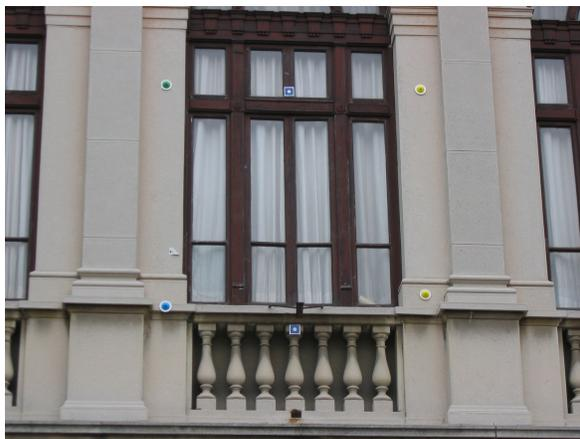
Figure 8. Targets acquired in both scans
