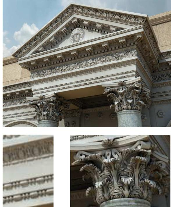
Figure 12. Second pediment from the left. The figure also shows some additional ornamental motifs, including the Corinthian capitals. Close-ups are shown in the bottom two images.
