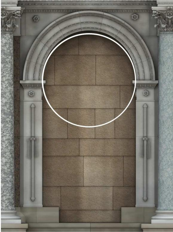
Figure 16. The arch above the third niche (from the left). The deviation from perfect circularity is clear.
