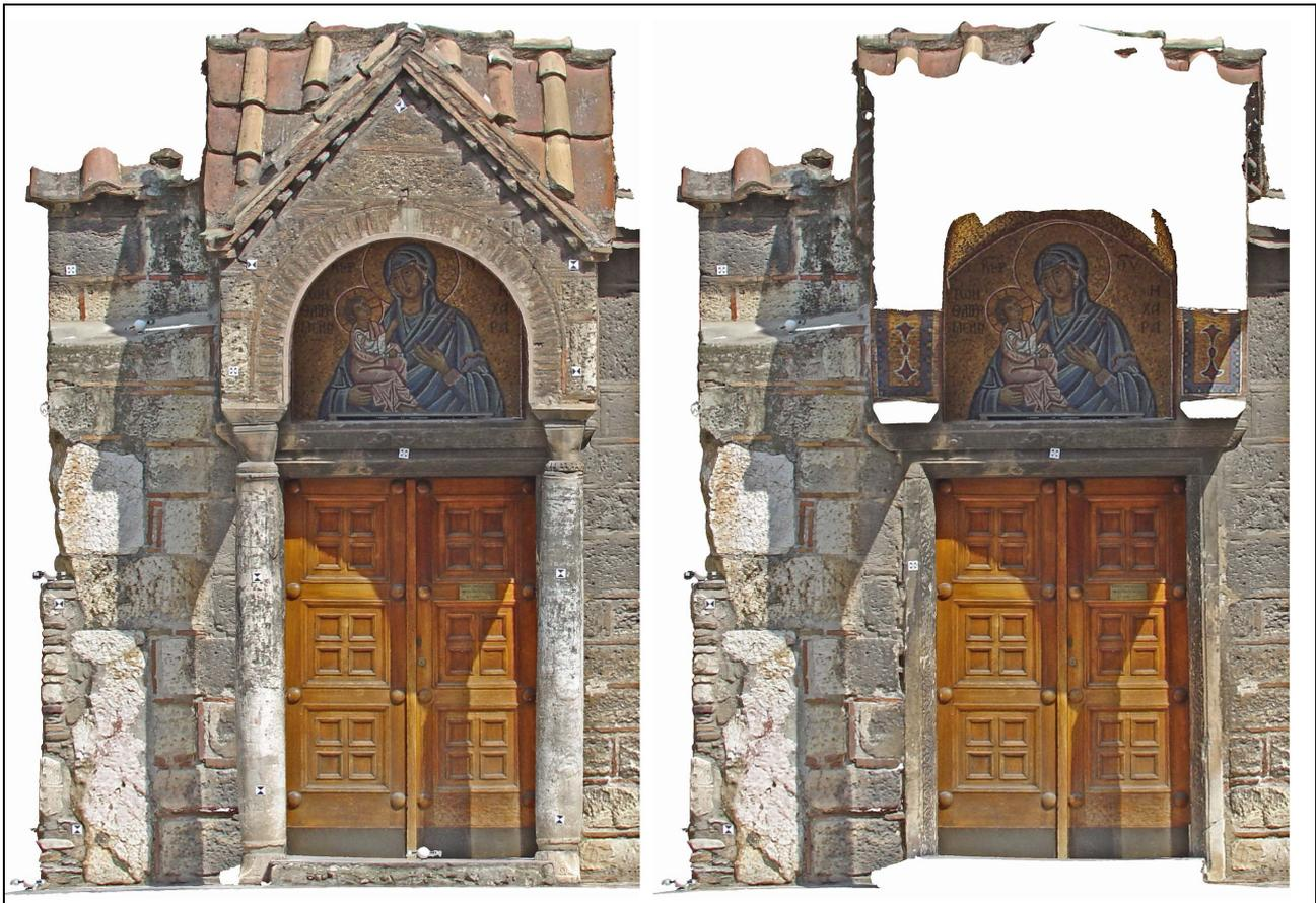
Figure 6. Left: Extract of the orthoimage from 7 images. Right: orthoprojection of a model section defined by a maximum Z-value.
