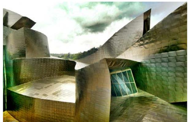
Figure 5 – The exterior panelling in tiles of titanium helped in the selection of the observed point coincident with the vertices and with the edges of the buildings
