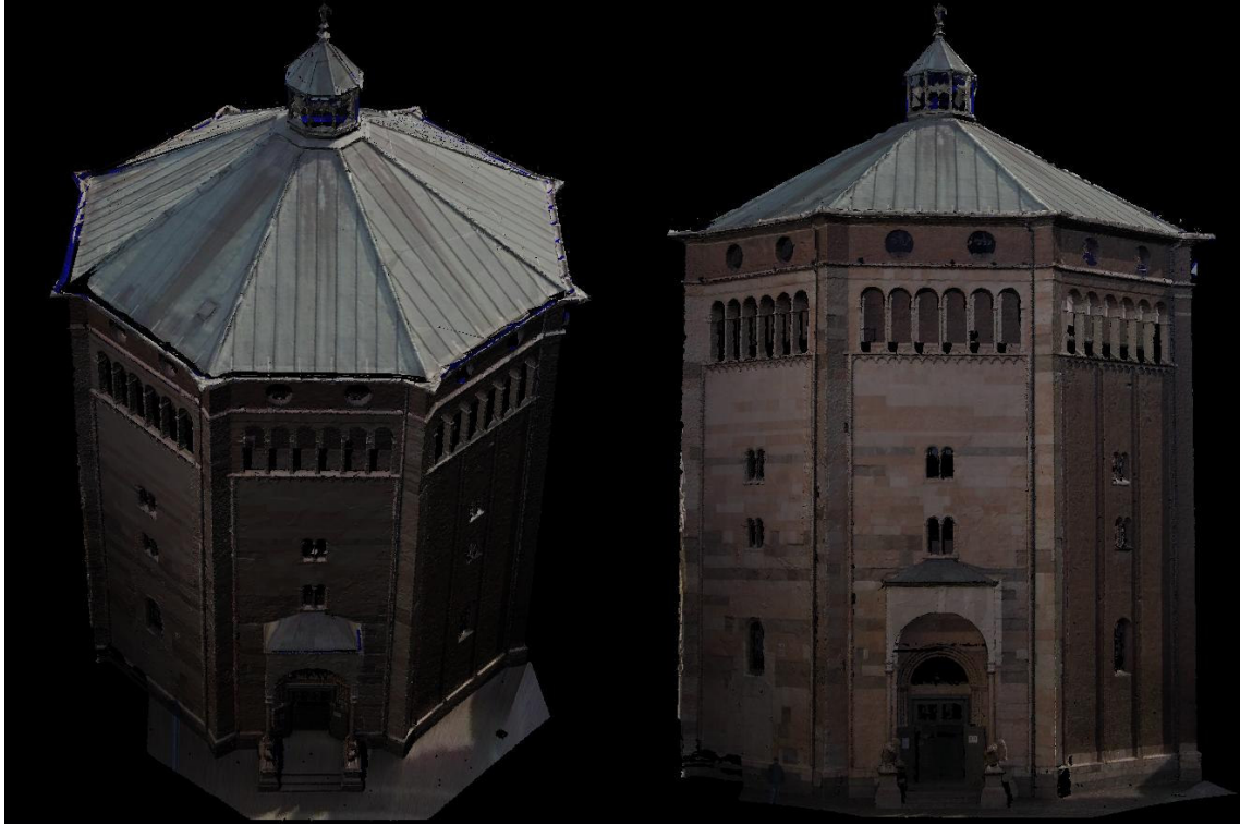
Fig 7 – Texture mapping of the North side of the Baptistery
