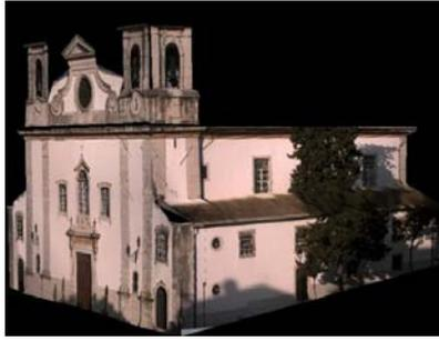
Figure 7. Perspective SW of the 3D model of the Oeiras mother church, rendered with rectified images
