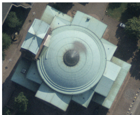
Figure 13. Complex roof structures (aerial image)
