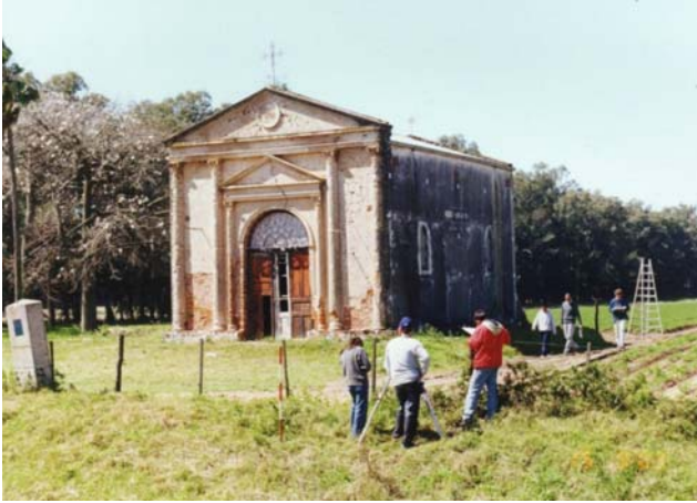
Figure 1. Saint Anthony's chapel façade
