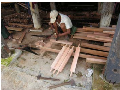
Figure 6. Renovation works at Shwei Yan Pye Kyaung
