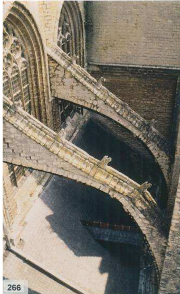
Figure 1: Outside the church: strengthening of buttresses, author.
