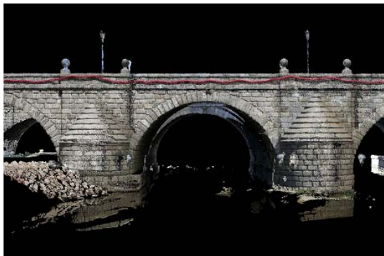
Figure 7: Puente de Segovia, M30 (Madrid, Spain).
