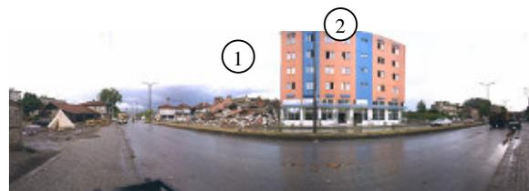
Figure 2. Panoramic QTVR views of the centre of Golcuk. Two identical buildings, 1 and 2, are showing a different resistance to shaking (QUEST).
