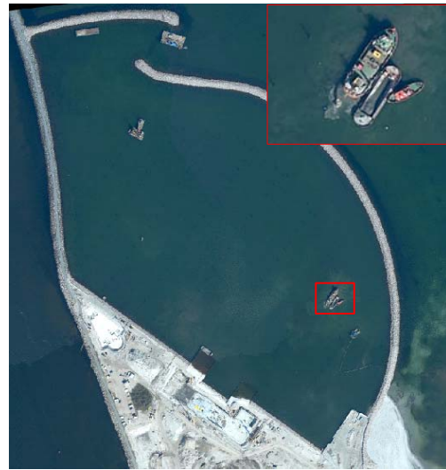
Figure 7: Harbour construction, 14.4.2004, 16 cm GSD, mosaic of 12 images, covered with PFIFF
