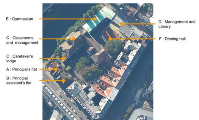
Fig. 9. Aerial view of “Pontonniers International High School” area in Strasbourg
